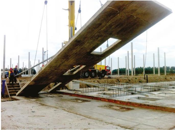
FIG. 8.2. Tilt-up panel (Source: own elaboration, 2018)
