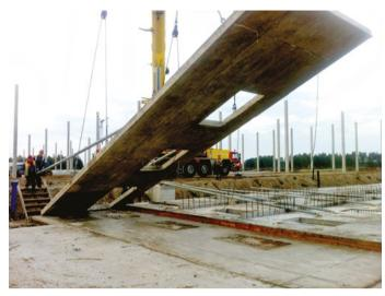
FIG. 8.2. Tilt-up panel (Source: own elaboration, 2018)
