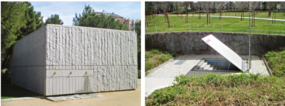
FIG. 4.10. Madrid-Rio Project, small objects located in the new public space, in Madrid, Spain. Left: Infrastructure and fountains with granite stone. Right: Emergency exit from underground tunnel (Source: photos by M a A. Flórez de la Colina, 2019)
