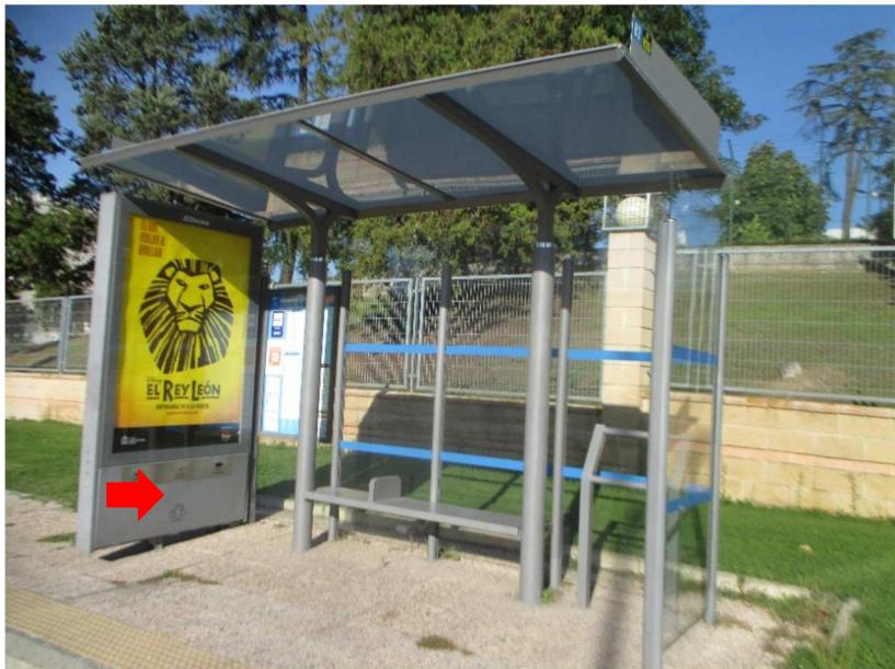
**Figure 11.** Bus Stop shelter with different types of battery containers on the lateral side.
