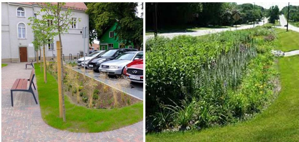
**Figure 2.** Bioretention trenches: a) Park in Górzycy (Photo: Anisko Architektura Krajobrazu), b) Greendale, Wisconsin, USA, (Source: WEB-1, 2021)
